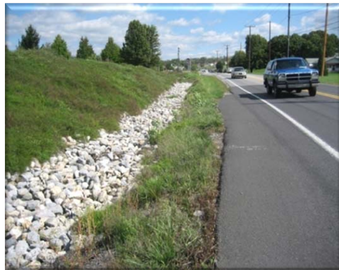
Rock-lined swale along site frontage
