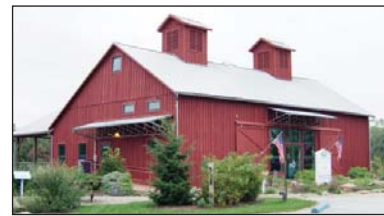
The Westmoreland Conservation District headquarters (1880s and 2001) – a 125-year-old, 7,600-square foot barn adapted with a variety of energy-conservation measures and used as the offices and education center of the Westmoreland Conservation District.
