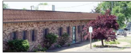
The Westmoreland County Public Works Building (1970) – home to the Westmoreland County Bureau of Parks and Recreation.
